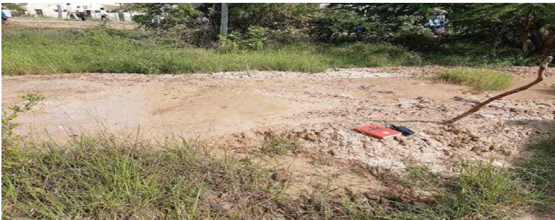
Picha Na. 28: Eneo la Kunduchi lililo bubujika tope ( liquefaction )
